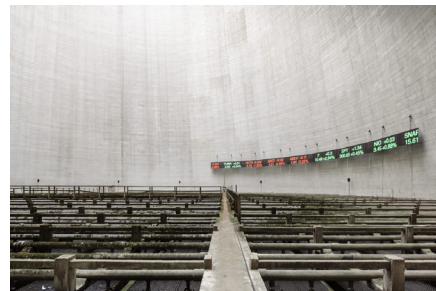
↑ Recoding the Existing Cooling Towers
