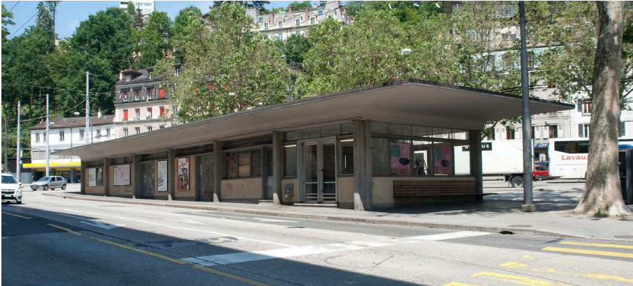
Figure 56. The old bus station
