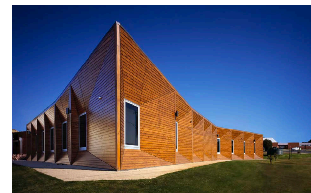
Figure 16. The facade following surrounding architectural style
