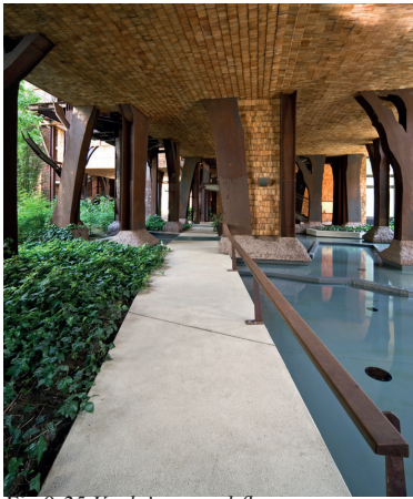
Fig.9 25 Verde's ground-floor water storage © Beppe Giardino
