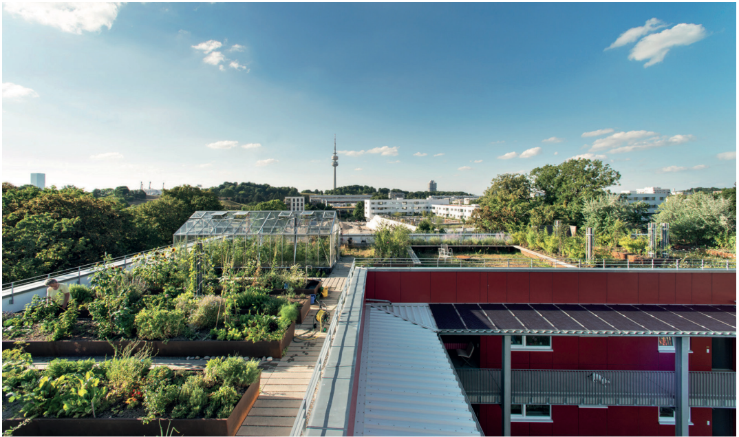
Fig.8 Wagnis 4 green roof view © Bernhard Rohnke
