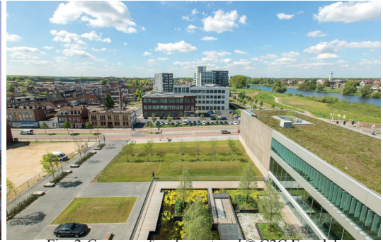
Fig. 2 Green roof and courtyard © C2C Expolab
