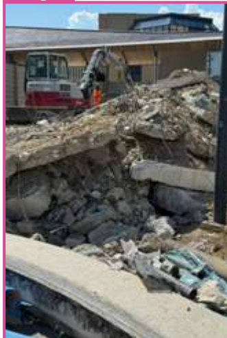
concrete from esplanade
