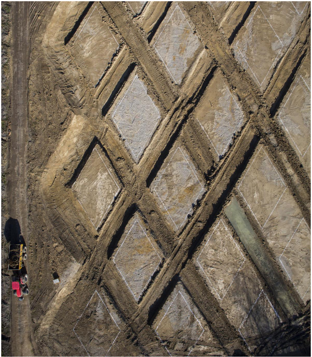
Renaturalization of the Aire river, the chocolate plate morphologie, photo by Fabio Chironi
