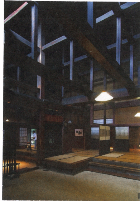
Yoshinuma's Doma Looking to (left to right) Daidokoro (family room), Nakao (inner foyer), DC (foyer).
