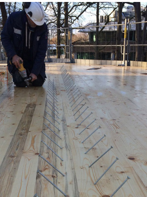
fig. 69 fixing the wooden structure (source: RAU Architects)
