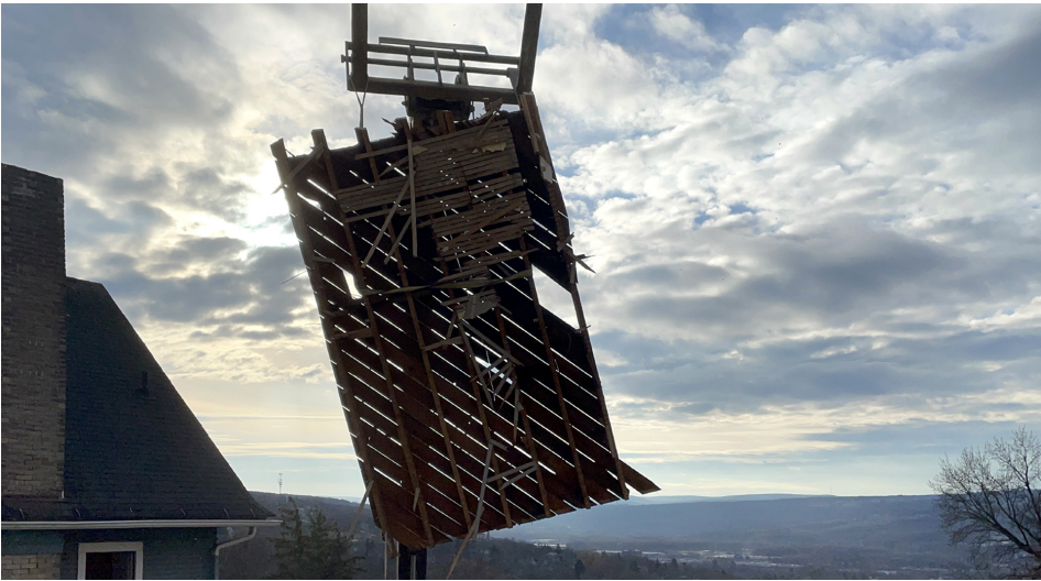
fig. 31 panelled deconstruction (source: photo credit: Felix Heisel)
