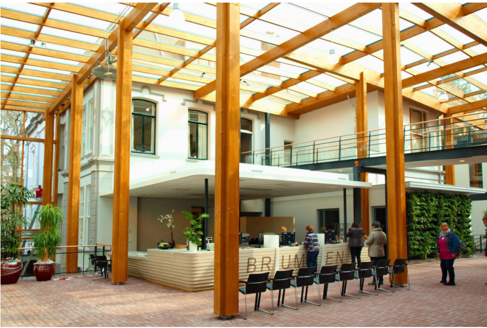
fig. 65 view on the inner courtyard and the demountable wooden structure (source: architectuur.nl)
