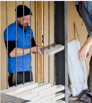
fig. 42 brick wall constructed without mortar (source: EMPA)
