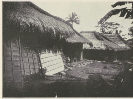
Figure 19. — A house complex prior to improvement.
