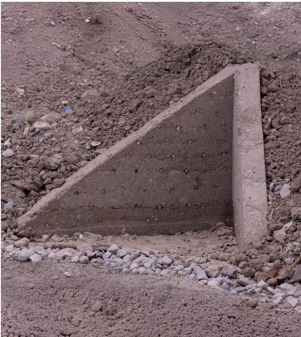
Rammed earth wall with wooden structure inside
