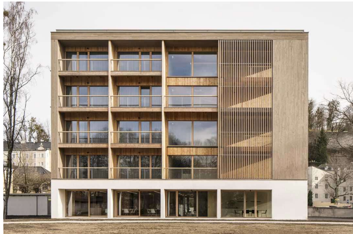
LP Architektur - RMD children's home 2021 - Salzburg
