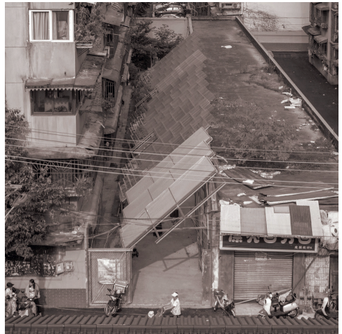
Yiie Arcitects – CACP “Designing?” in Yulin Second Alley, Chengdu City, China (2024)
