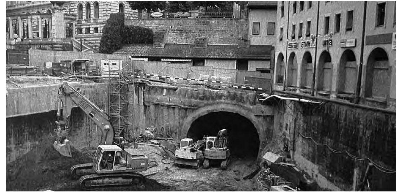
Image: Construction of the M2 tunnel in La Riponne, c. 2004.
