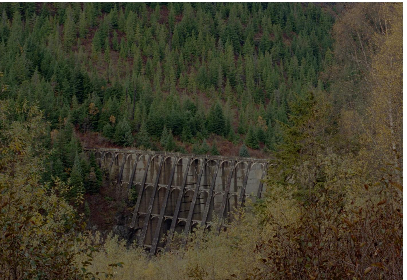
All that is now left at the site of the old town, are the concrete storage dam - which was breached when the Anyox was abandoned - a massive tailings pile of copper ore slag, and the foundations of several crumbling buildings.
