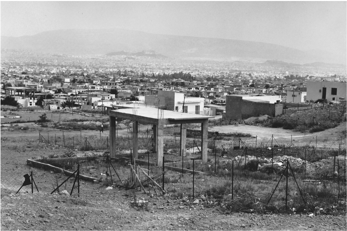
Unauthorized construction in reinforced concrete with protruding rebar over the roof slab. © Aristides & Maria Romanos, Architectural Association
