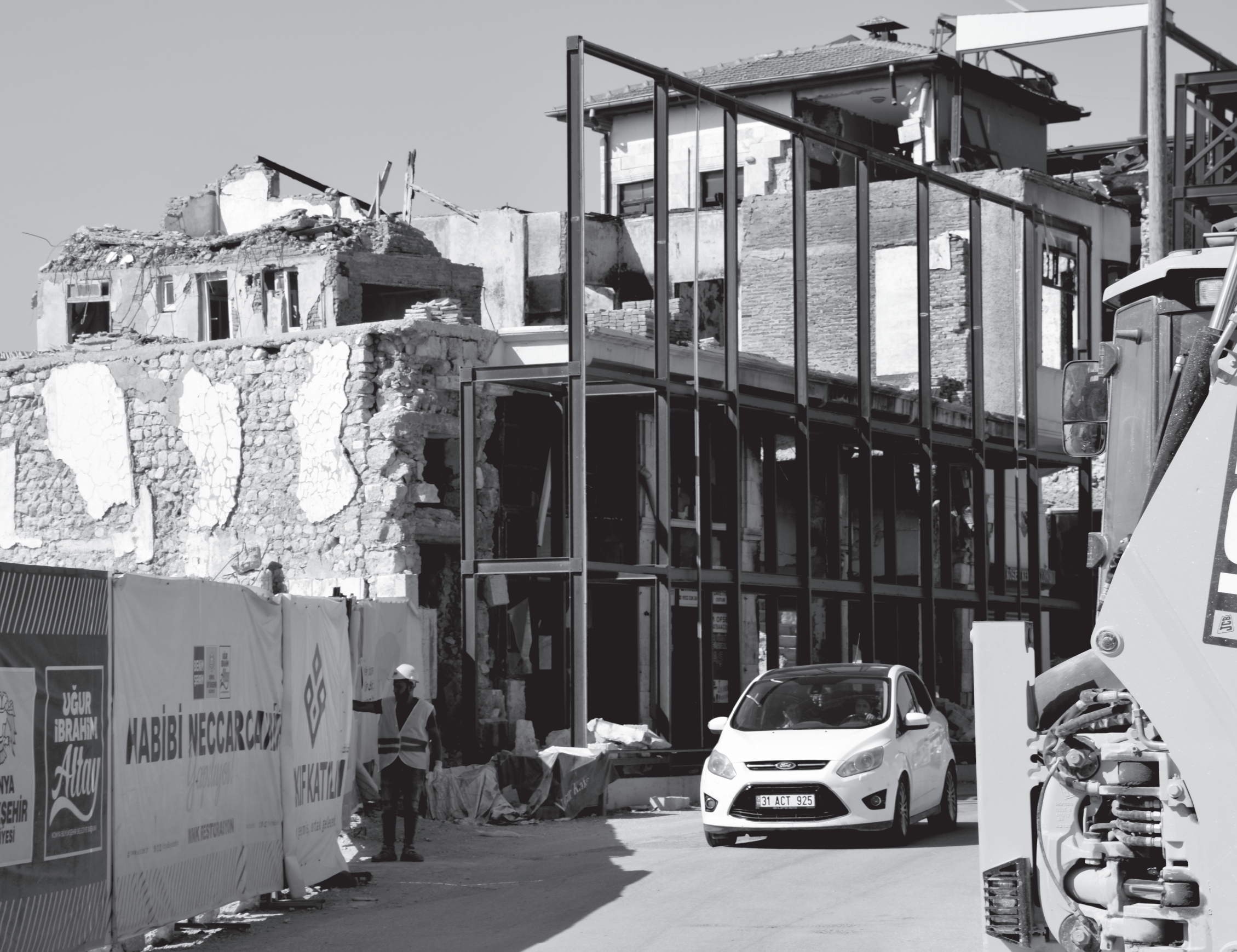
Fig. 24: Efforts to preserve the historic building supported by scaffolding, August, 2024.
