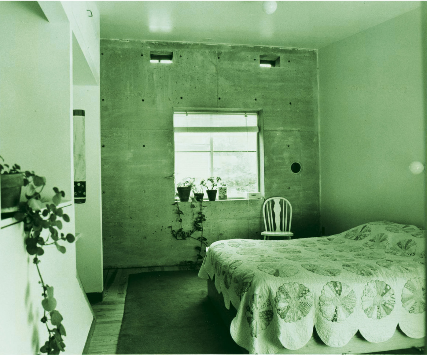
Fig. 9: Interior view of the Trombe wall from the bedroom (Source: Kelbaugh, D., 1975)
