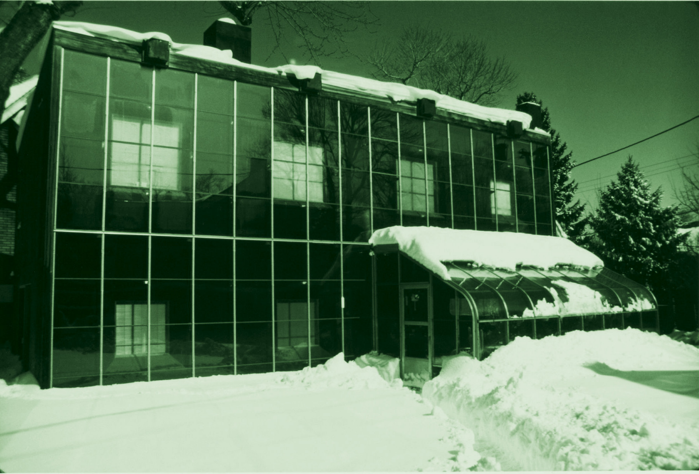
Fig. 8: Exterior view of the Trombe wall and greenhouse (Source: Kelbaugh, D., 1975)
