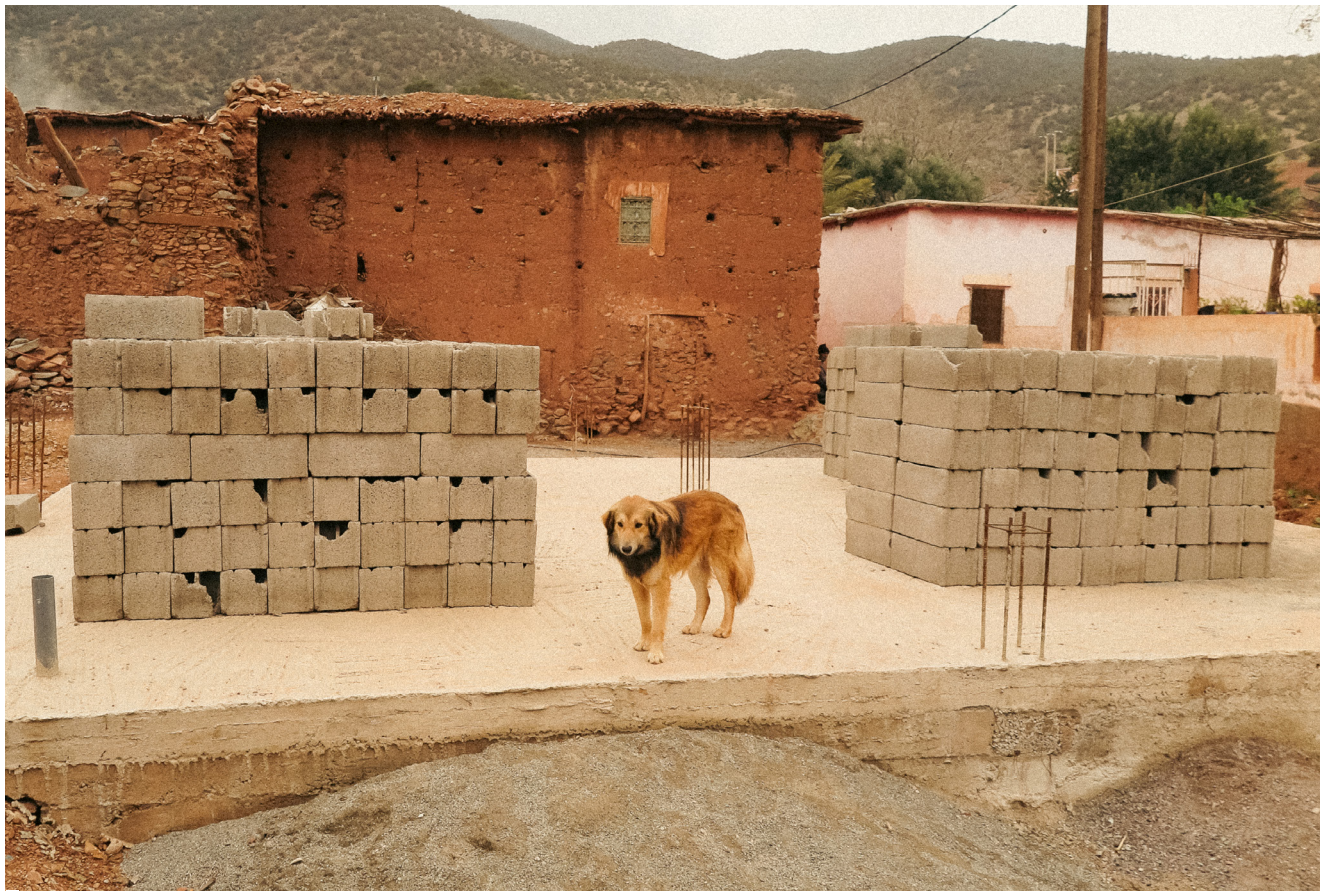
From earth to concrete Ouirgane, March 23, 2025
