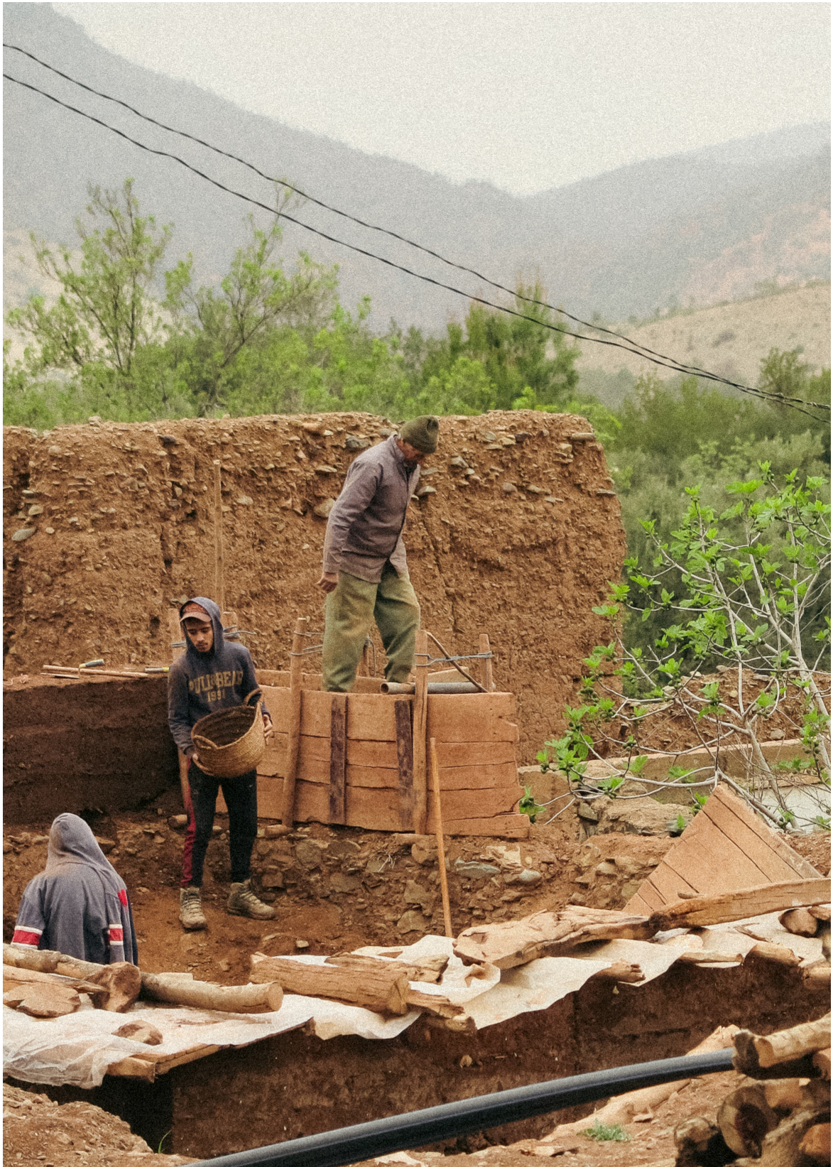
Rammed earth construction with traditional formwork, involving coordinated roles: carrying, filling, compacting Quiqane, March 23, 2025
