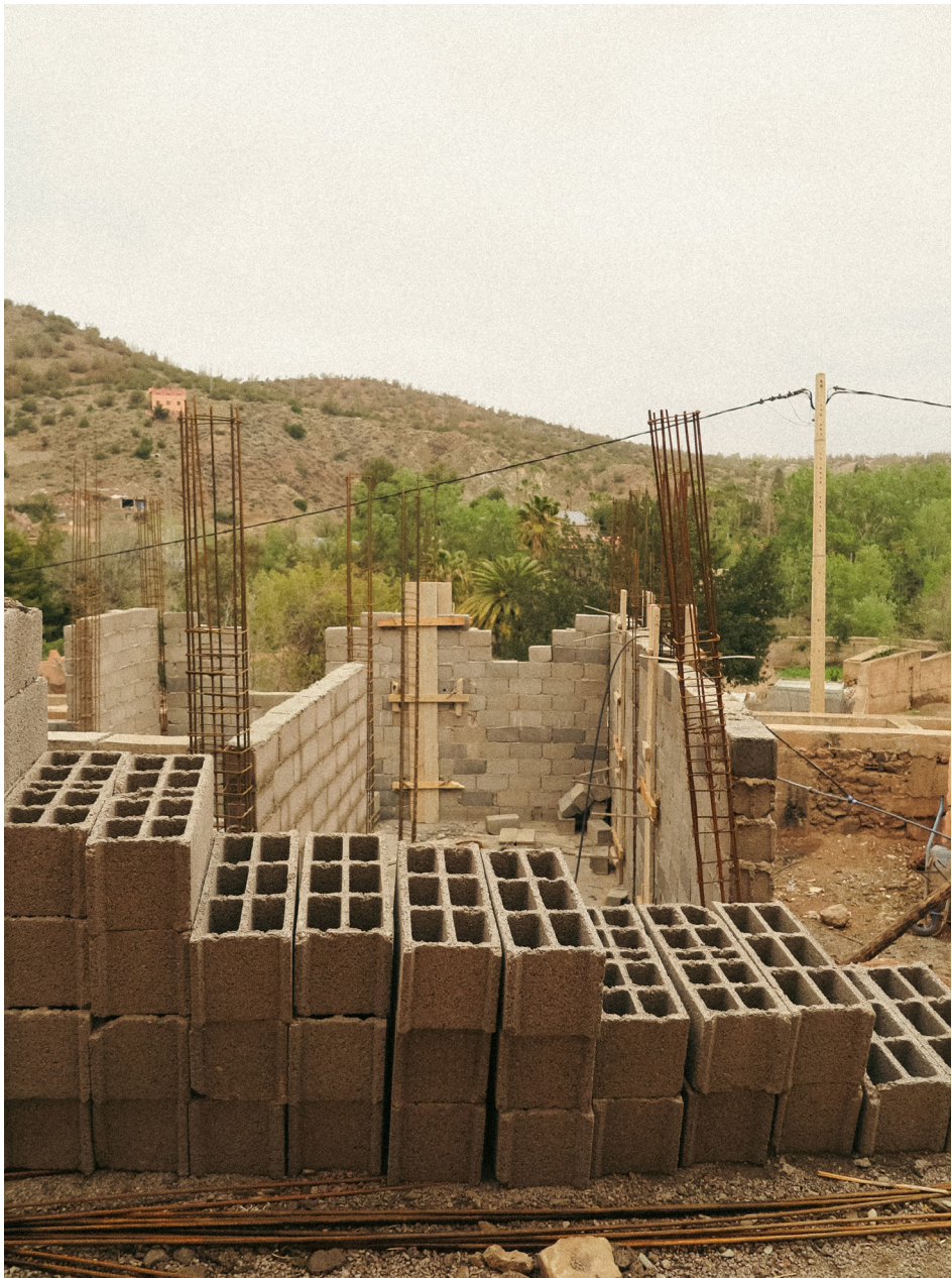
Reconstruction : Wall construction Ouirgane, March 23, 2025
