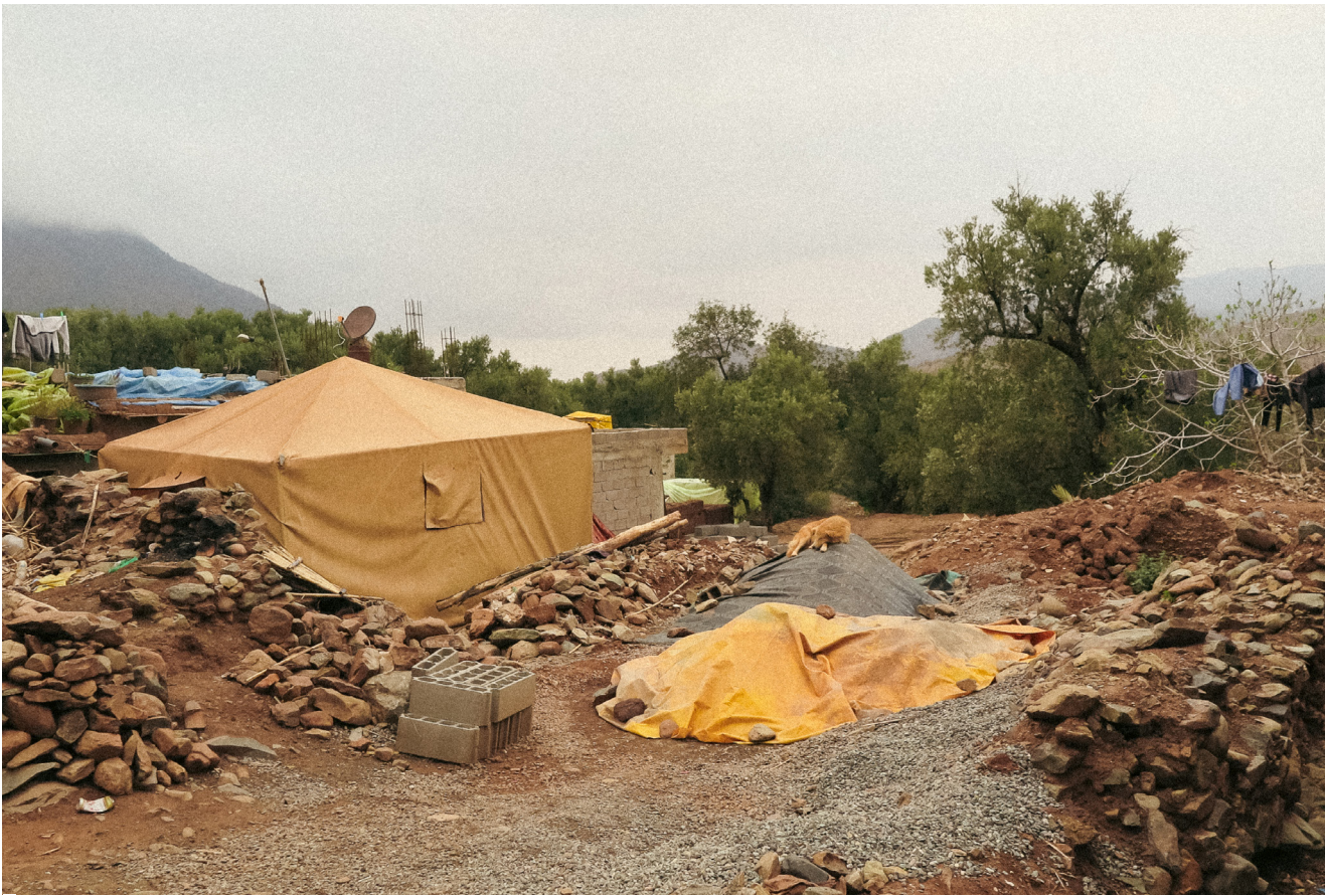
Temporary shelter coexisting with ongoing reconstruction efforts and material storage Ouirgane, March 23, 2025
