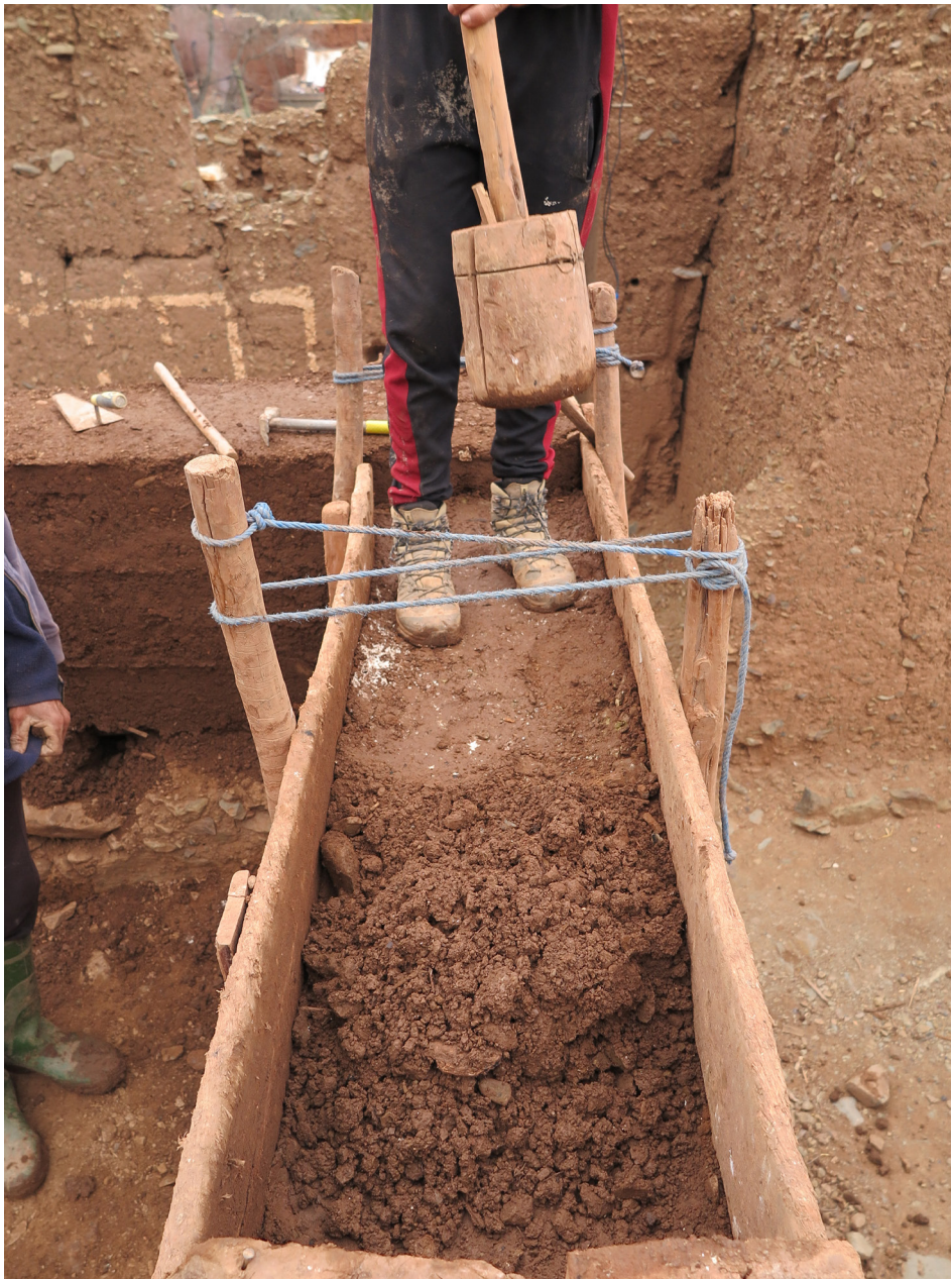
Earth compacted in layers using a wooden rammer Ouirgane, March 23, 2025
