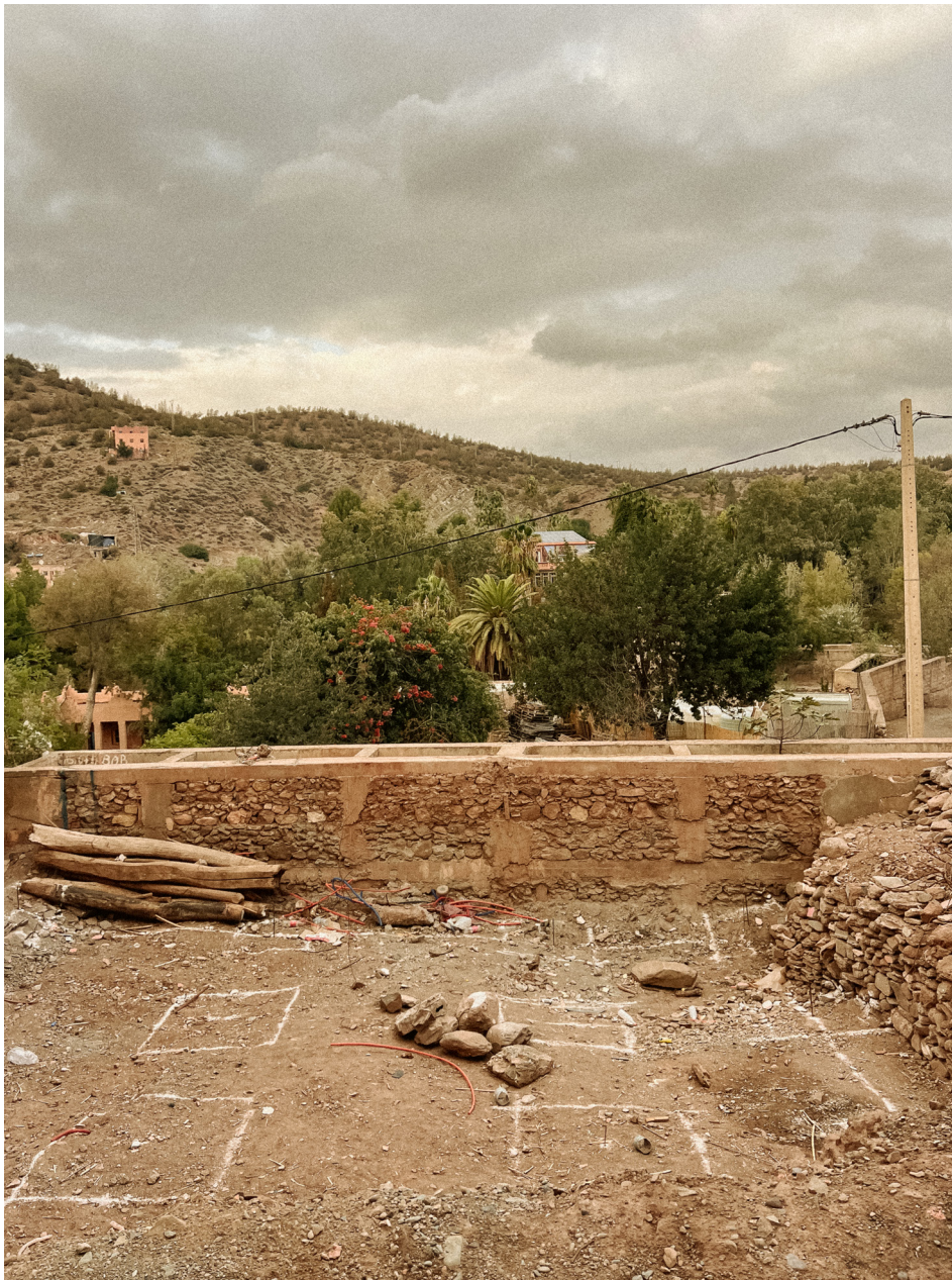
Reconstruction : Ground marking before digging Ouirgane, October 14, 2024
