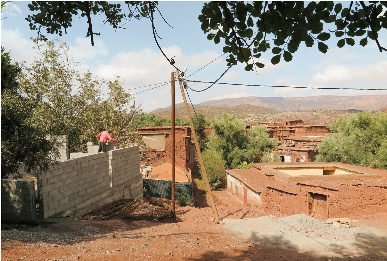
Concrete rising over earthen traces Ouirgane, October 14, 2024
