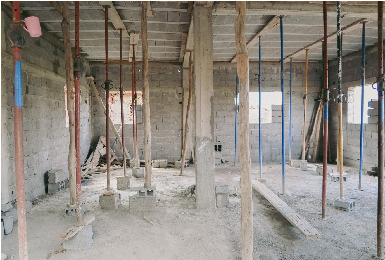
Interior of a typical reconstruction house in progress Ouirgane, October 14, 2024
