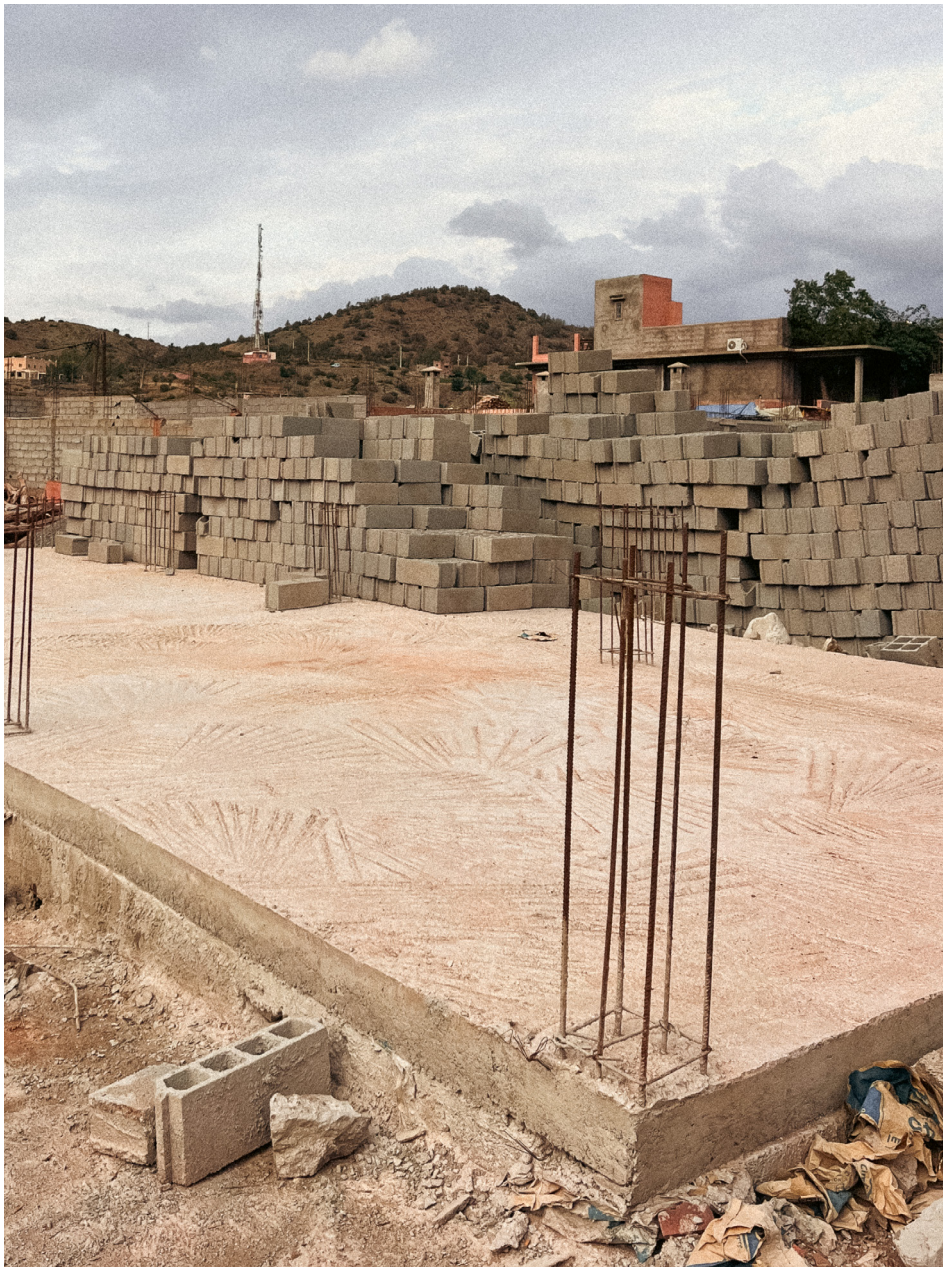
A typical site using reinforced concrete and hollow concrete blocks as default materials for reconstruction Ouirgane, October 14, 2024
