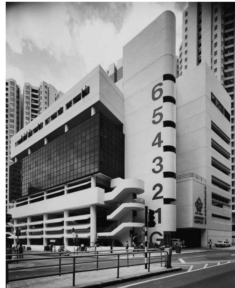
Fig 3.2.21 Aberdeen Municipal Service Building achevé en 1983. Source: Dennis Lau & Ng Chun Man Architects & Engineers (HK) Limited, "Exterior Photograph, Urban Council Aberdeen Market Complex (circa 1979-1983), Aberdeen, Hong Kong" M+ Collections.
